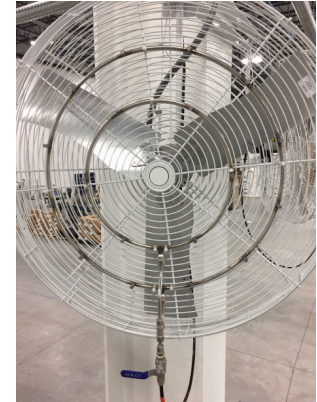
Figure 7 — 36" fan with mist ring
