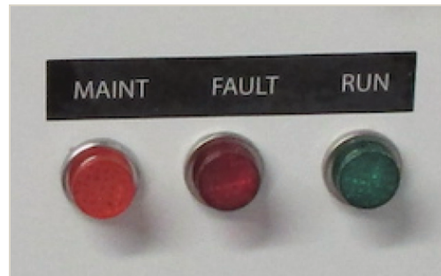
Figure 5 — Indicator lights: MAINT (amber, 500 hours), FAULT (red, pressure not proven), RUN (green, pump on).
