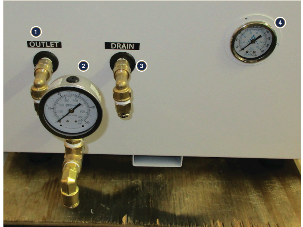
Figure 2 — Front view, water facilities end.
