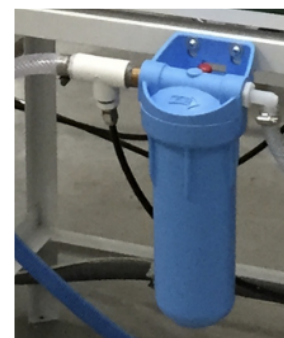
Fig. 12.2 5-MICRON SEDIMENT PRE-FILTER Cartridge Filter Housing, Part #92609
