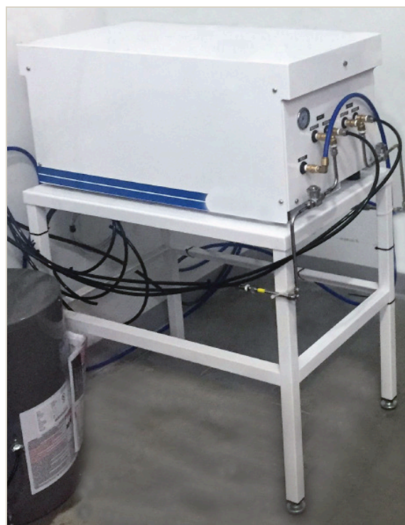
The FanMist Automated Pump Station: pump, controls and safety systems in one enclosure.
