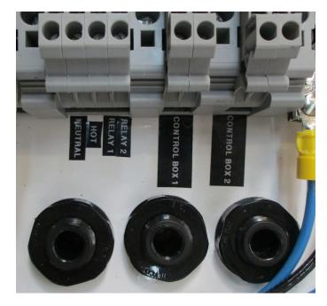
Connect Humidistat Terminal #8 (marked Humidify contact output) for Zone #2 to internal connection marked Relay 2 (This is where the incoming 24VAC Hot from the Neptronic should land in order to activate Zone #2).
