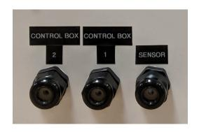
All 24VAC Fan Control Wiring for each zone is routed through the corresponding label CONTROL BOX 1 for Zone 1, CONTROL BOX 2 for Zone 2 (where the 24V wiring will be sleeved, to send the 24VAC signal to the fan relay boxes).
